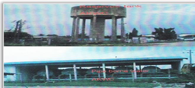
Figure 5: Akwa Ibom Water Corporation (AKWC) reservoir tank and pipe borne water treatment facility about 18 metres away from septic tank
