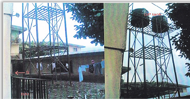
Figure 2: Borehole located 4.2 metres away from septic tank at a premises located along Akpan Essien Street
