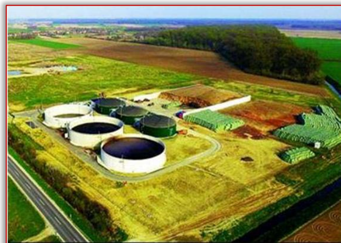
Figure 4. Biogas power plants (2 MW) "Biointegra" Slatina, Croatia [8]
