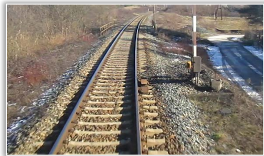
Figure 7. Position of rail balize.
