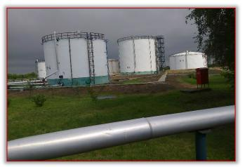
Figure 3. The appearance of the oil collecting station The process of extracting crude oil from gas can also begin in the collection pipelines itself specific pressure and temperature of the mixture. In the collection stations, the units are separated gas is extracted from crude oil. Then the butane and propane, carbon dioxide are separated from the gas obtained and sulfur.
