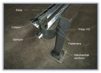
Figure 4: The semi heavy restraint system studied
