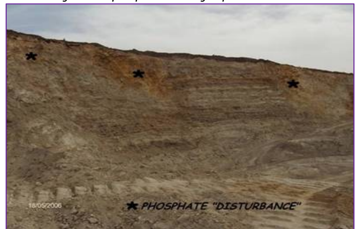
Figure 2. Example of "disturbance" affecting the phosphate strates. The hardpan pockets are normally detected only at the time of drilling. Direct exploration methods such as well logging or surface geology are not particularly effective.
