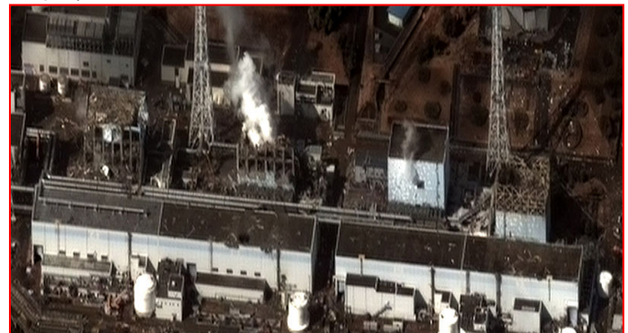
Figure 3– Fukushima Daiichi nuclear disaster - four damaged reactor buildings [9].
