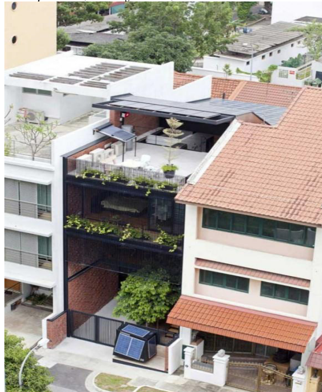
Figure 4. Building fixed with photovoltaic panels
