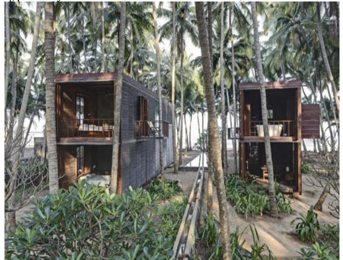
Figure 6. Palmyra house in India that utilizes a local aqueduct irrigation system with water harvested from four on-site wells
