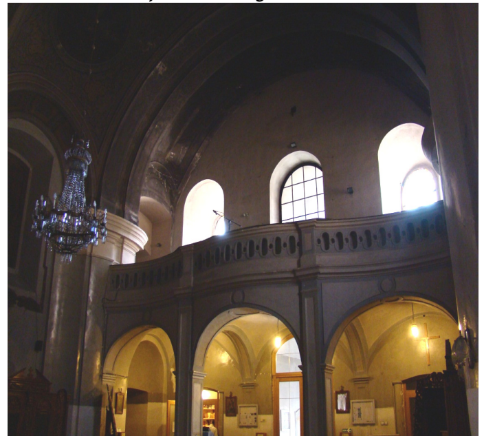
Figure 5. First vault segment
