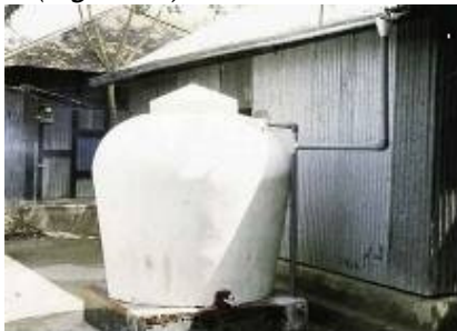
Figure 11. Ferrocement Rain Water Tank
