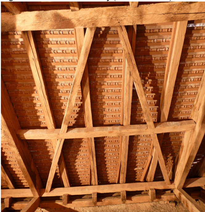
Figure 3. Crossbars in the rafter section
