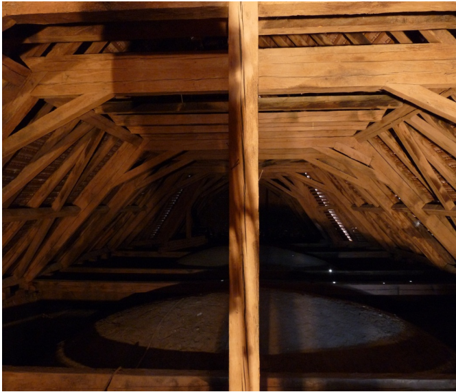
Figure 1. The roof framing
