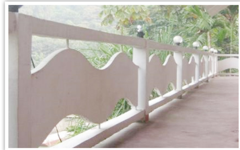
Figure 4. Ferrocement for balconies
