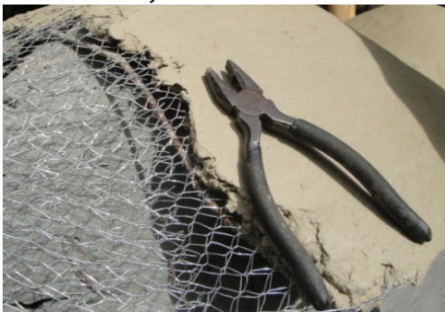
Figure 1. Ferrocement element
