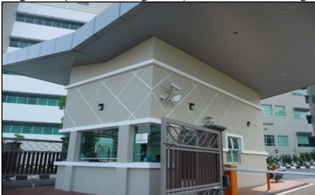
Figure 8: Pan Tilt zoom at the guard house in IPharm building
