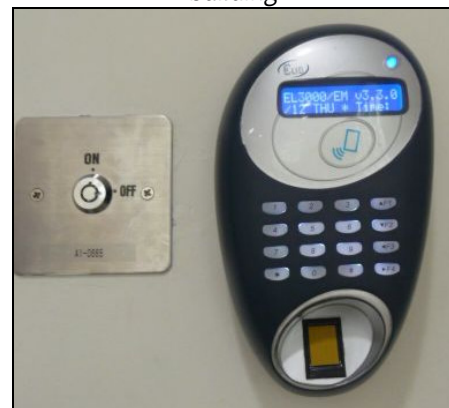
Figure 3: Thumb print access control system in Eureka building
