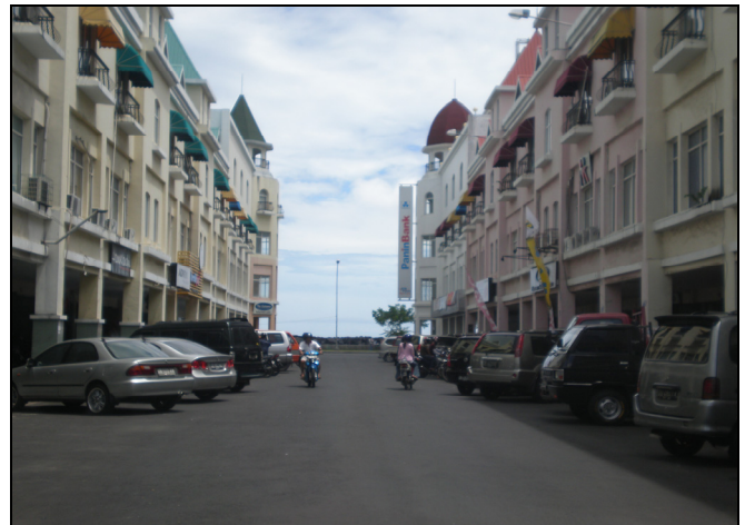
Figure 4. Stores and home office on the reclamation Area
