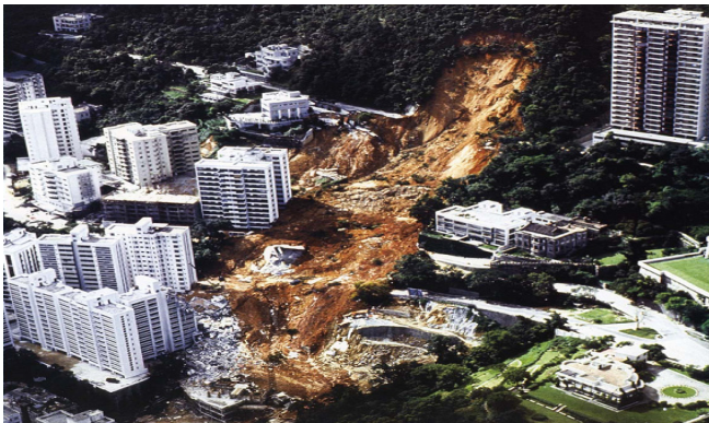
Figure 1. Landslide at Sau Mau Ping in 1976 [8]
