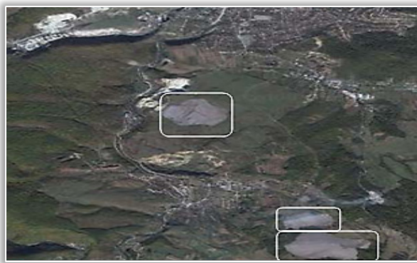
Figure 1. The tailings dams where the mining tailings (sideritic waste) were stored at Teliuc [2,4,12,15]
