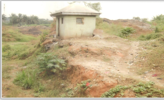
Figure 3: A gully in Uyo (near old dumpsite along Uyo village road), gradually becoming stabilized by vegetation cover. Source: Researcher.
