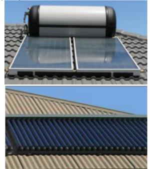
*Figure 1. Flat panel (left) and evacuated tube collectors i. Flat plate solar collectors*
