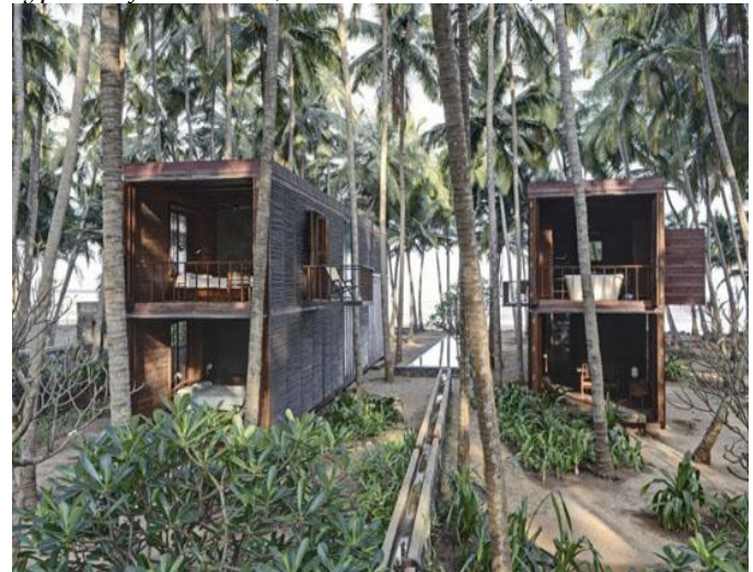
Figure 6. Palmyra house in India that utilizes a local aqueduct irrigation system with water harvested from four on-site wells
