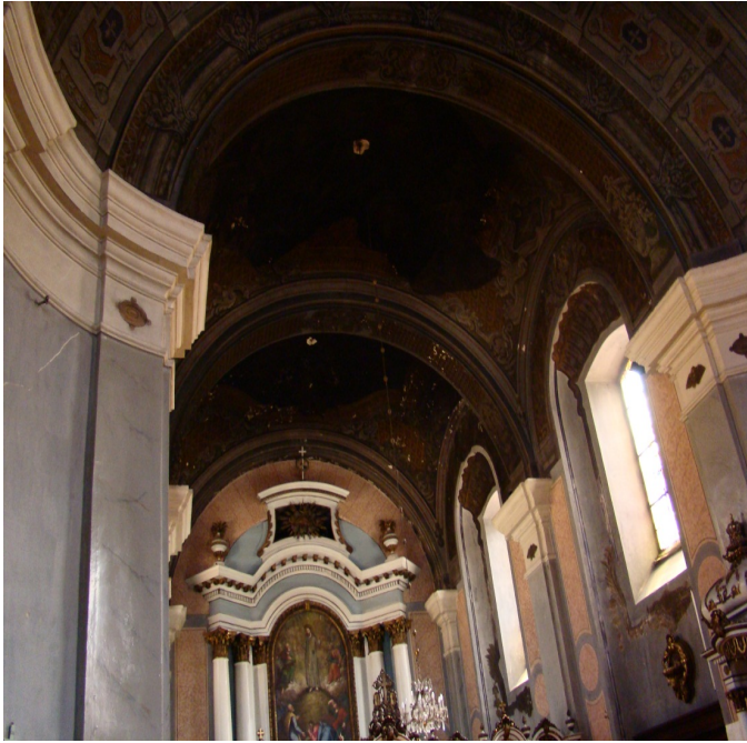
Figure 6. Suspended domes with rectangular plane geometry
