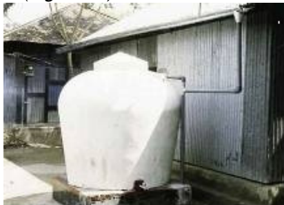
Figure 11. Ferrocement Rain Water Tank
